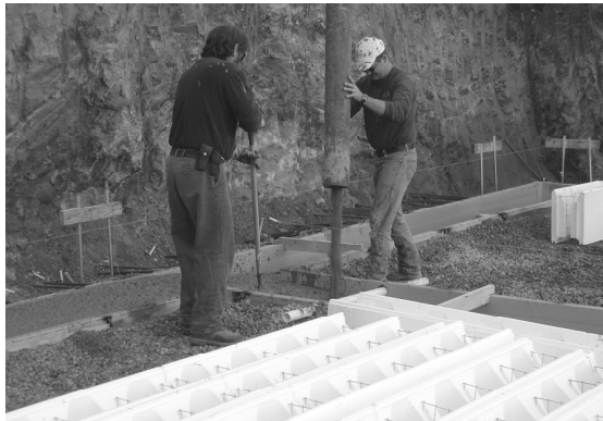
CONSTRUCT A LEVEL FOOTING
