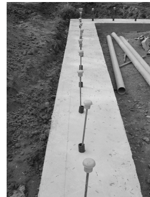
CONSTRUCT A LEVEL FOOTING
