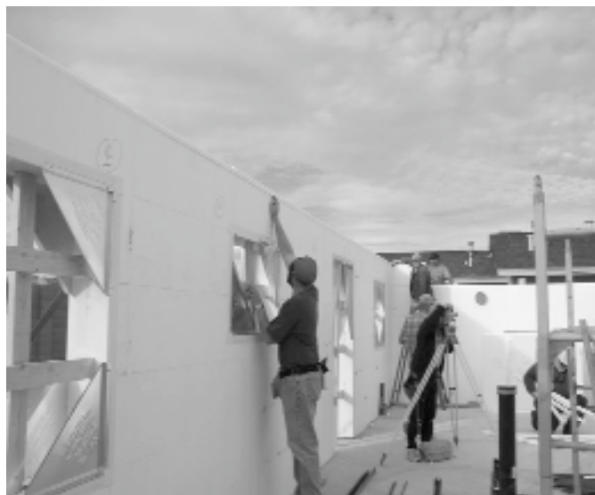
SNAP A LINE TO MARK THE PLATE HEIGHT AND MARK FORMS FOR PLACEMENT
