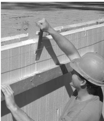
SIMPSON HANGER INSTALLATION
