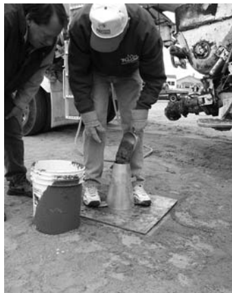
PLACE CONCRETE IN CONE
